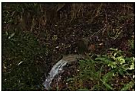
Photo 39 : Stormwater pipe outlet on western part of De Mond
