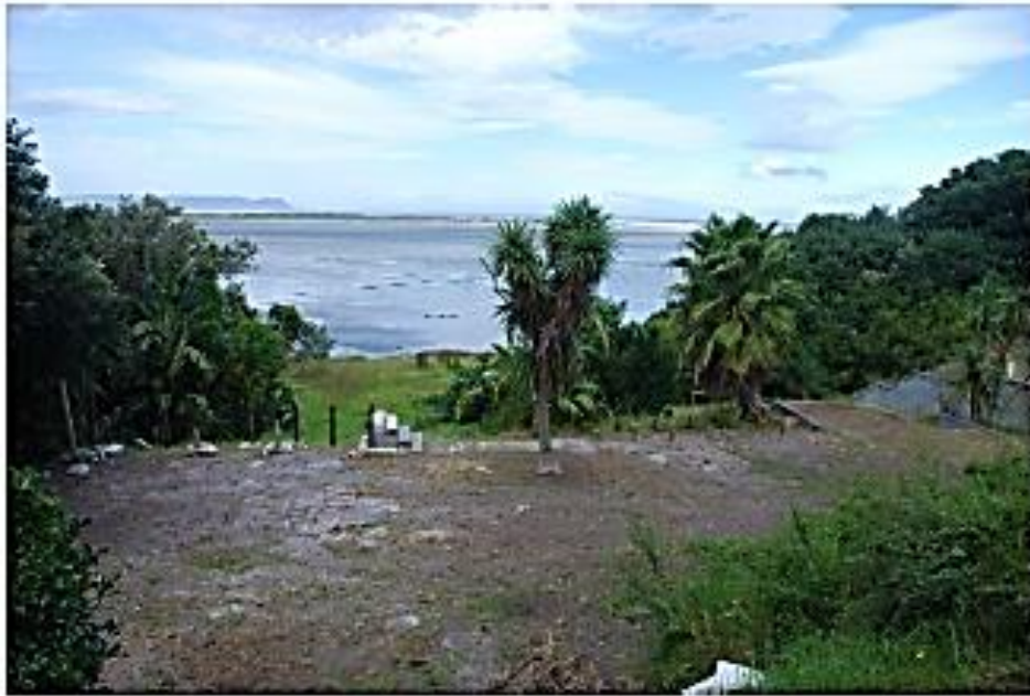
Photo 11: One of the vacated stands at the De Mond Caravan Park. This terrace is above the 5 m contour. A more environmentally friendly and aesthetic gravity retaining wall system should be used in the re-development of the Caravan Park. The alien trees and shrub species should be removed. The lower terrace could be rehabilitated using indigenous grasses for use as a public open space.
