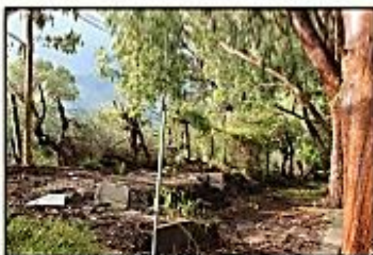
Photo 60 : Condition of boundary fence along the R43
