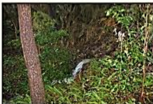
Photo 38 : Stormwater pipe outlet on western part of De Mond
