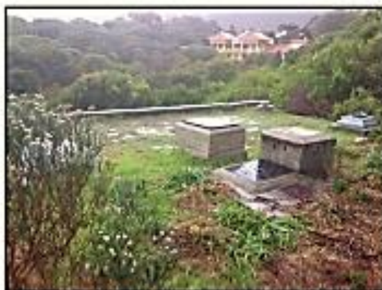
Photo 71 : Mosselriver sewage pumping station : Roof of pumping station
