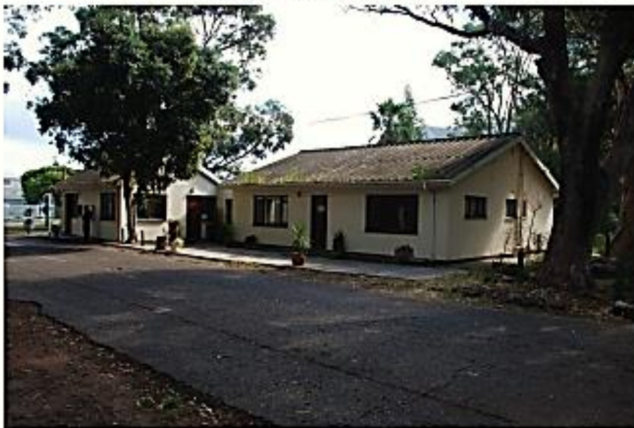
Photo 1: Views of the existing controlled access point into the De Mond Caravan Park from the suburb of Voëlkop to the west. Note the security and office building. These buildings could be refurbished and retained.
