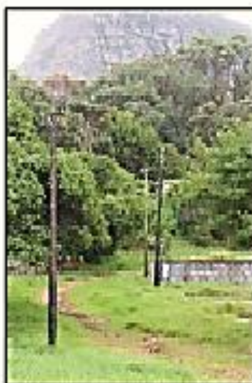
Photo 52 : Overhead electricity cables at De Mond
