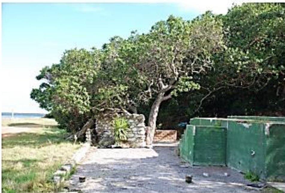
Photos 21 and 22: Vacated stands at the De Mond Caravan Park. These stands, and others like them, should be completely cleared of building materials and foundations, and rehabilitated under the supervision of an appointed ECO and Landscape Architect. The Milkwood Trees especially must be protected from disturbance when existing concrete foundations, paving and slabs / floors are removed. Removal of such structures around the trees should be undertaken by hand.
