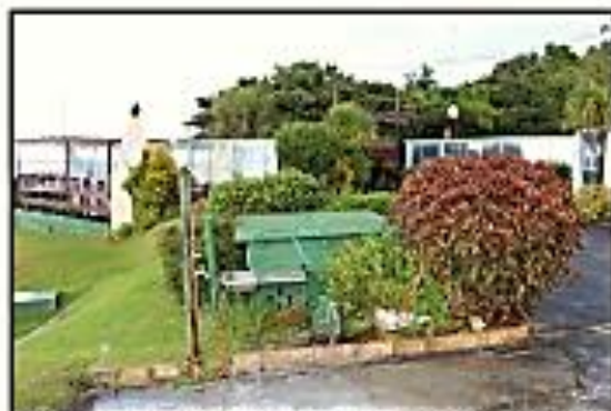
Photo 32 : Sewage collection point (conservancy tank) at Klein River Lagoon Park
