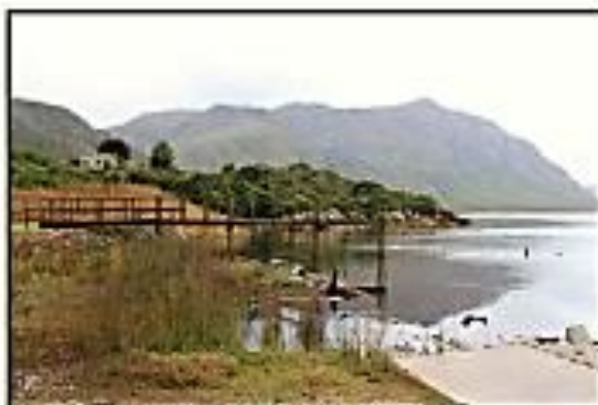
Photo 18 : Existing Jetty at Prawn Flats
