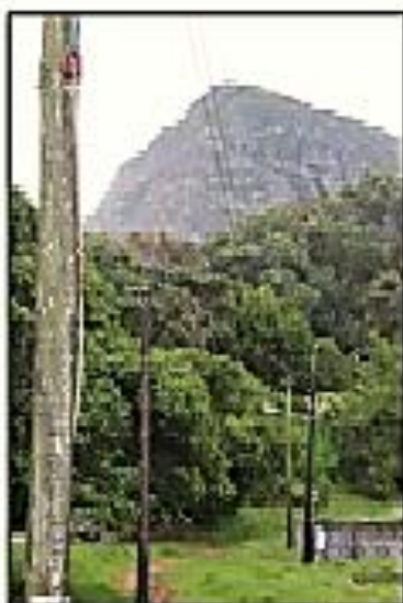
Photo 51 : Overhead electricity cables at De Mond
