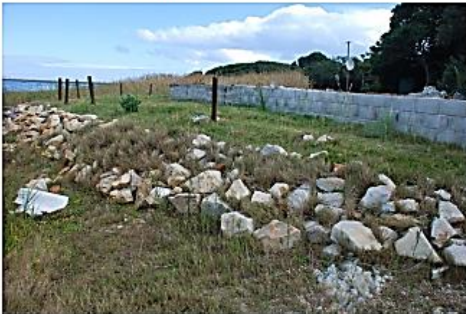
Photo 20: One of the vacated stands at the De Mond Caravan Park. This stand, and others like it, should be completely cleared of building materials and foundations, and rehabilitated under the supervision of an appointed ECO and Landscape Architect. The rock revetment, used to protect the structure, should also be removed.
