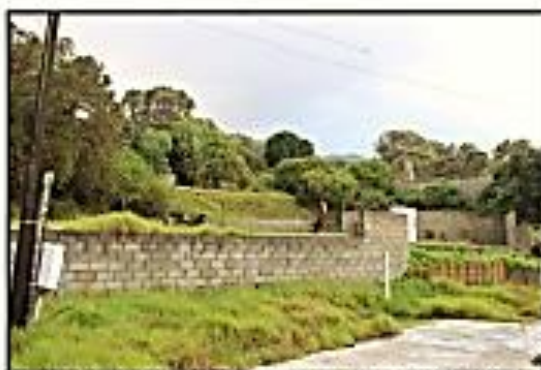
Photo 50 : Existing retaining walls at De Mond
