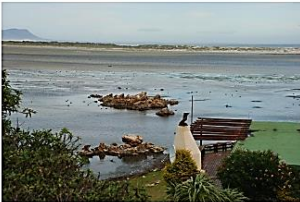
Photo 7: View from the De Mond Caravan Park over a “park home” at the Klein River Lagoon Park. This “park home” and others are situated below the 5 m set-back level for the lagoon should therefore be removed.
