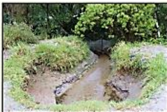
Photo 16 : Stormwater channel above Klein River Lagoon Park
