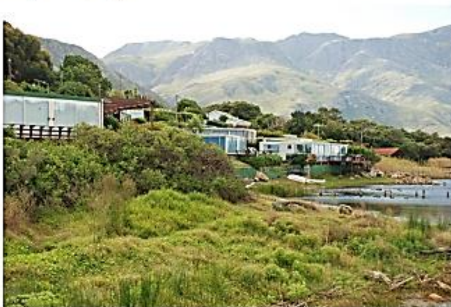
Photo 18: View along the estuary margin towards some of the existing houses at the Klein River Lagoon Park. These houses are situated between a mixture of indigenous and exotic garden tree species. The retaining wall is built of concrete blocks and is probably at a height of ± 2.5 m. This retaining wall should be removed and a more environmentally friendly sea-wall constructed (such as a waterlöffel gravity retaining wall system). This wall can be terraced towards the resort to a height of ± 3.2 m above mean sea level (i.e. above the natural breaching level of the sand berm across the estuary mouth).
