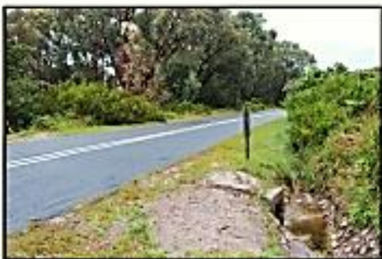
Photo 11 : Stormwater culvert crossing of R43 near Prawn Flats access
