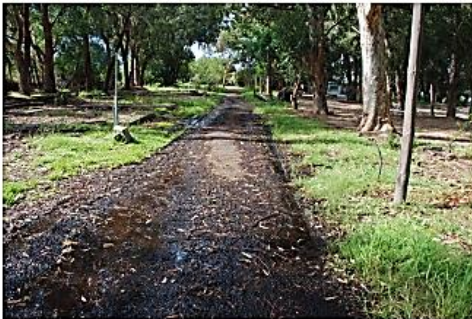
Photo 3: View to the east along one of the internal roads in the De Mond Caravan Park. This road is located on the northern side of the property. This surface wetness is likely to be as a result of groundwater seepage flowing from properties to the north higher up the slope. An engineering solution will need to be found to deal with this seepage water, e.g. by constructing a cut-off drain along the northern boundary of the site.
