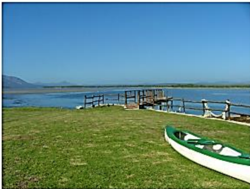
Photo 27: A grassed earth-rubble-filled terrace has been constructed at a height of approximately 2.8m above mean sea level at Prawn Flats to provide ease of access for the public to boats off a fixed wooden jetty. Even so, portions of the Prawn Flats recreational node and parking area are occasionally flooded when the estuary mouth is closed to the sea by a sand berm. A proper sea-wall should be built for retaining the fill of the grassed terrace. The jetty should also be reconstructed.
