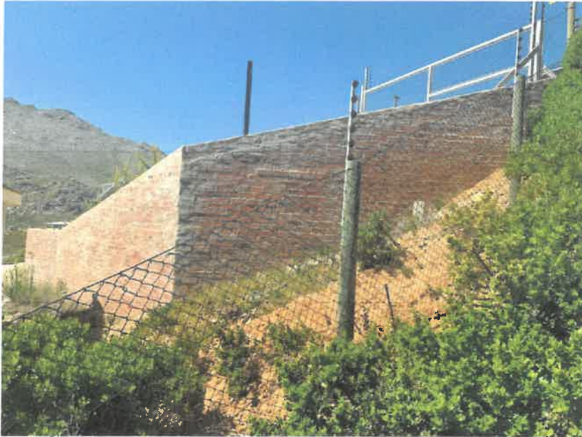
Neighbouring property (Erf 316) with garage lower down on Erf to accommodate the steep fall. The approach-driveway is constructed at +2m above NGL at it's highest point, inside the street building line, also due to the steep road embankment. Vehicle access to the plot would be impossible without fill. As a result of the long driveway here, extensive natural vegetation on the embankment have been sacrificed.
