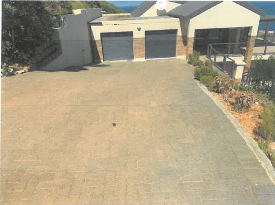
Neighbouring property (Erf 318) with garage on Roella Road Erf Boundary, with entrance parallel to Roella Road. Erosion and surface water run-off is problematic and much Fynbos have been sacrificed.
