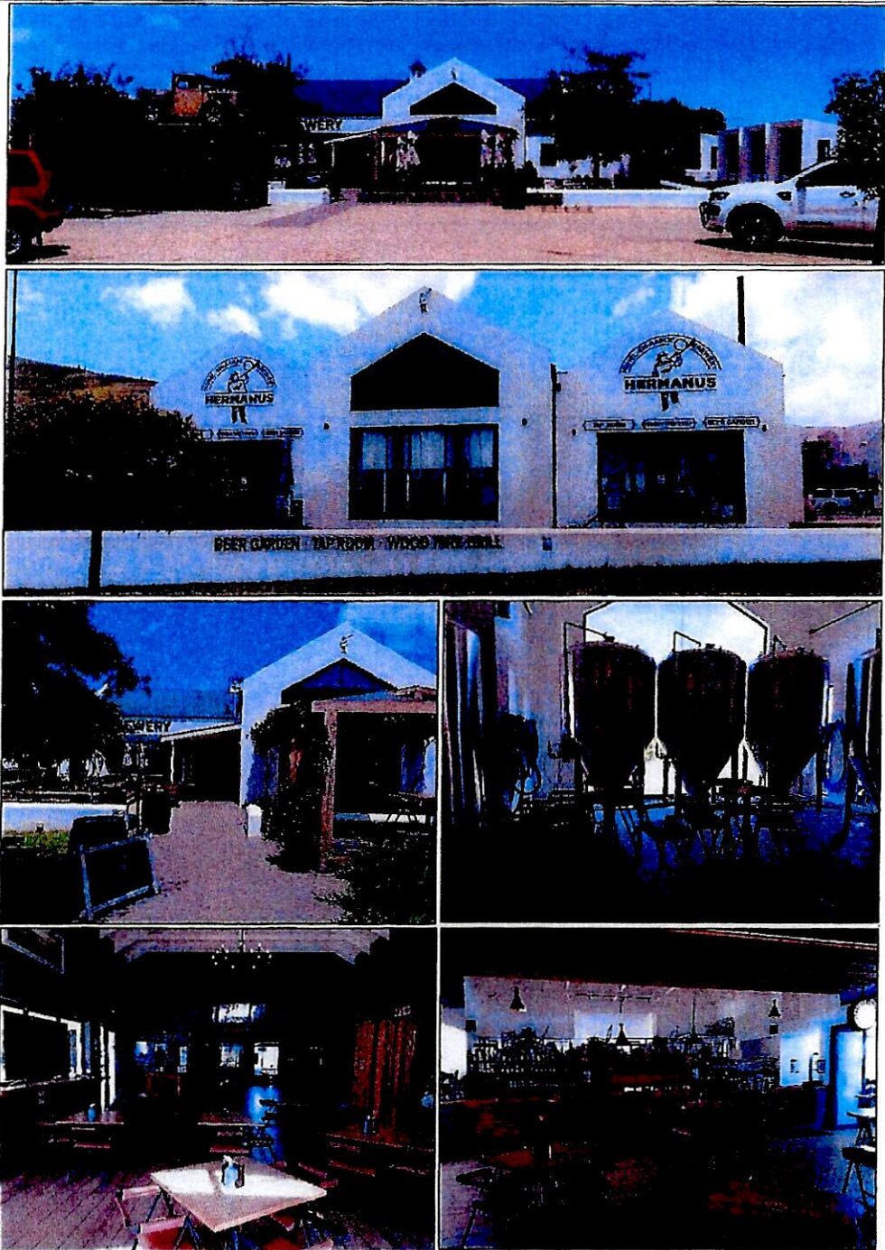
Figure 11: Photographs of the facilities on the application site
