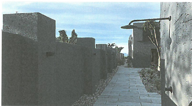
The North Eastern boundary wall with pillars that will support the proposed covered walkway
