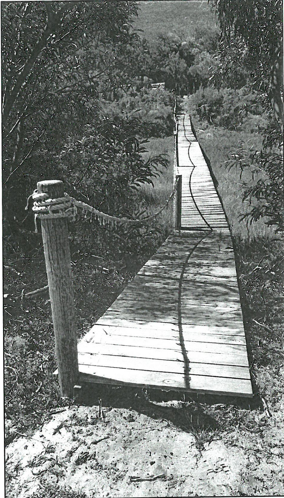
Photo 5: Existing bridge over water.
