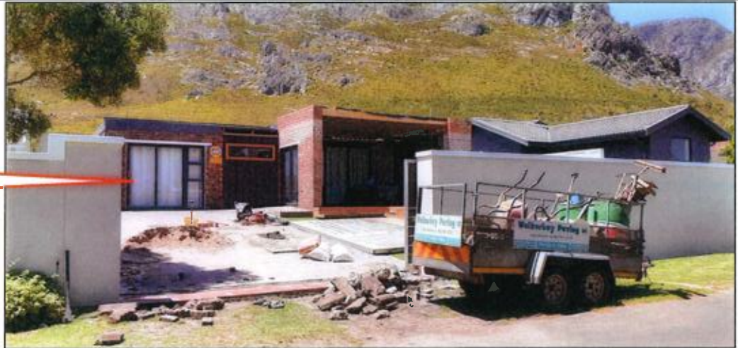
Figure 11: Front and Back Views of Existing New Guest Bedroom
