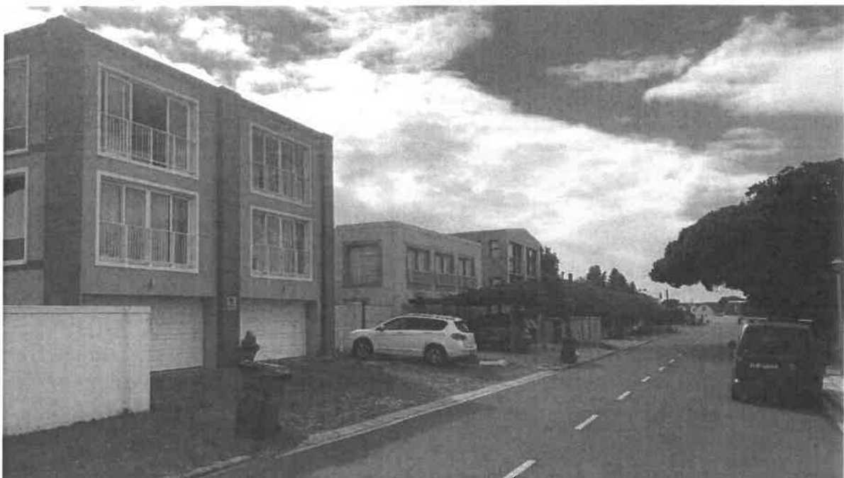
Figure 4: Looking east down Tenth Street with the property in question on the left after the three dwellings.
