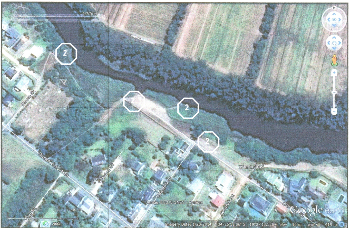
AERIAL PHOTO showing the location(s) of Node 2 where the abluent block, jetty, two walkways, resurfacing of access road slipway and parking area and bird hide will be.
