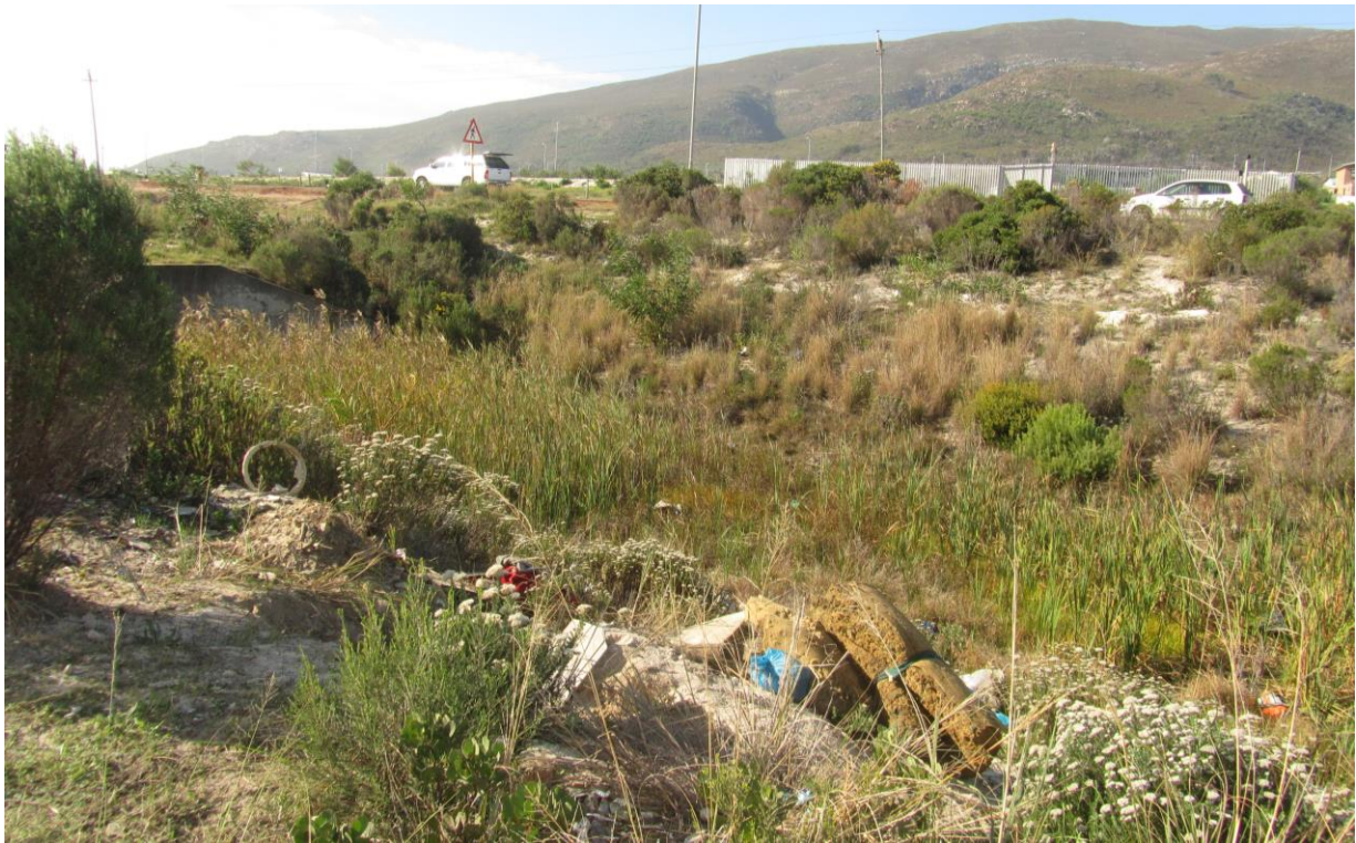
Plate 4: View of the stormwater attenuation adjacent to the R43 Road
