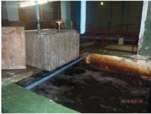
Gravity flow dosing system of flocculent
