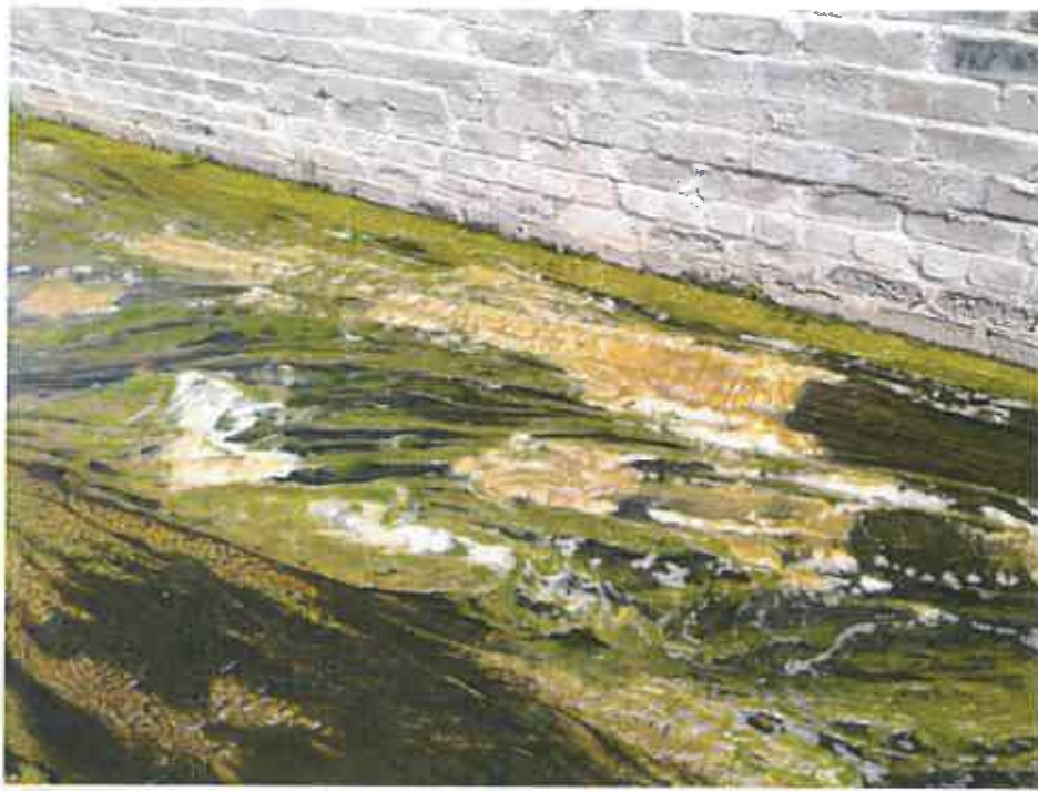
Figure 8A typical example of a concrete gully with algae growth
