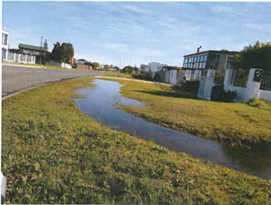
Figure 2 Indicating a lack of rain water drainage on the eastern side of Main road
