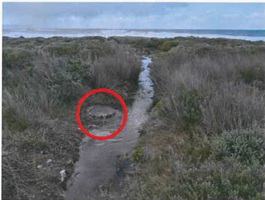
Figure 4 Note the excess water spillage from a sewer line during a downpour
