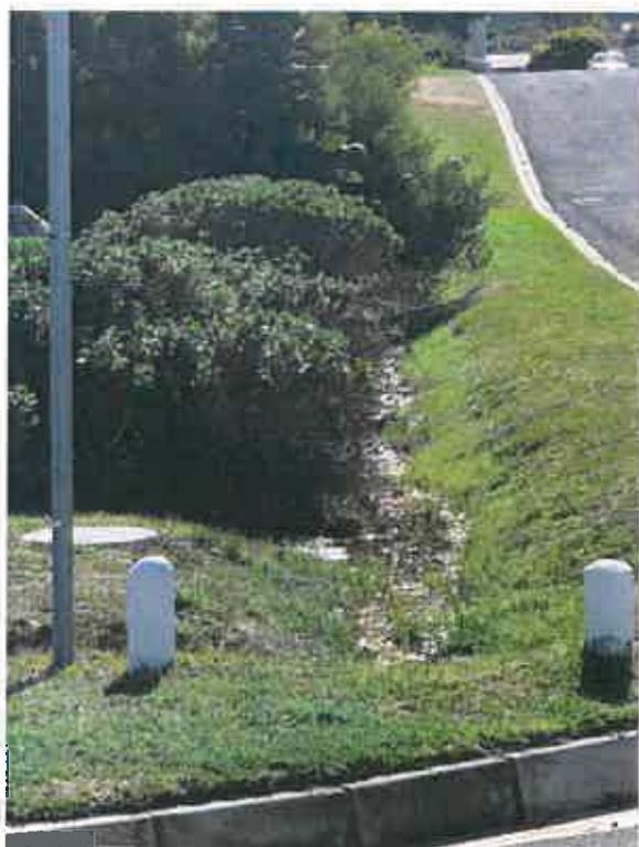
Figure 7 A typical example of a water gully in Sandbaai that is overgrown with vegetation
