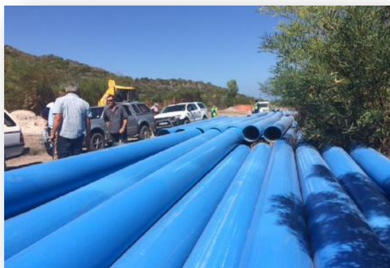
Construction of the new bulk water supply pipeline to Gansbaai
