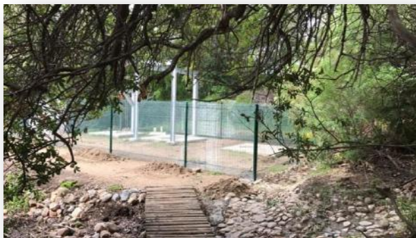
New sewerage pump station constructed at Stanford
