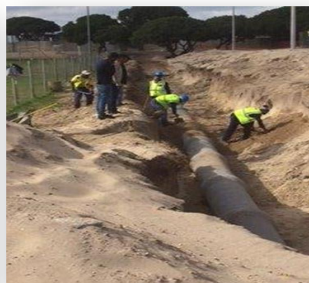
Construction of Storm water infrastructure, Masakhane, Gansbaai
