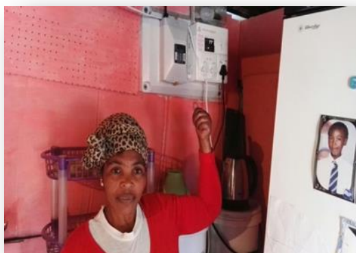
Electrification of informal housing in Thambo Square site
