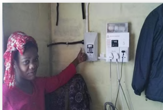
Electrification of formal housing in Admin site
