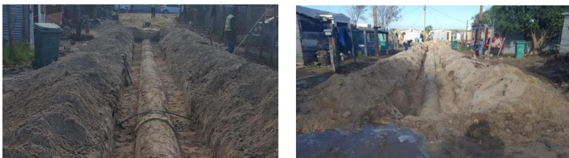
Bulk Sewer Pipelines, Zwelihle
