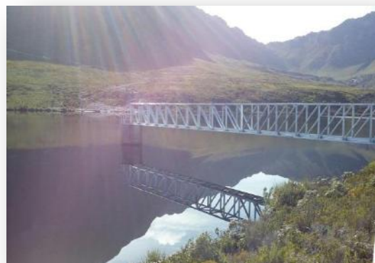
The new bridge at the intake tower of the Buffels River Dam
