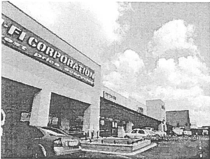
Stoneridge Shopping Centre, Edenvale.
