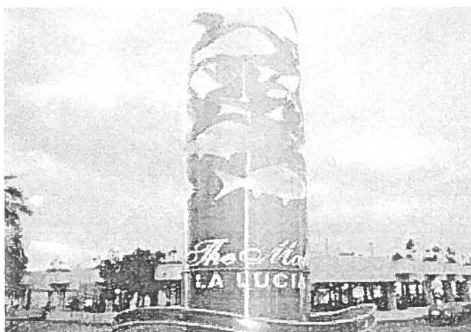
La Lucia Mall, Durban: A strong localised centre in competition with the larger super regional centre, Gateway.
