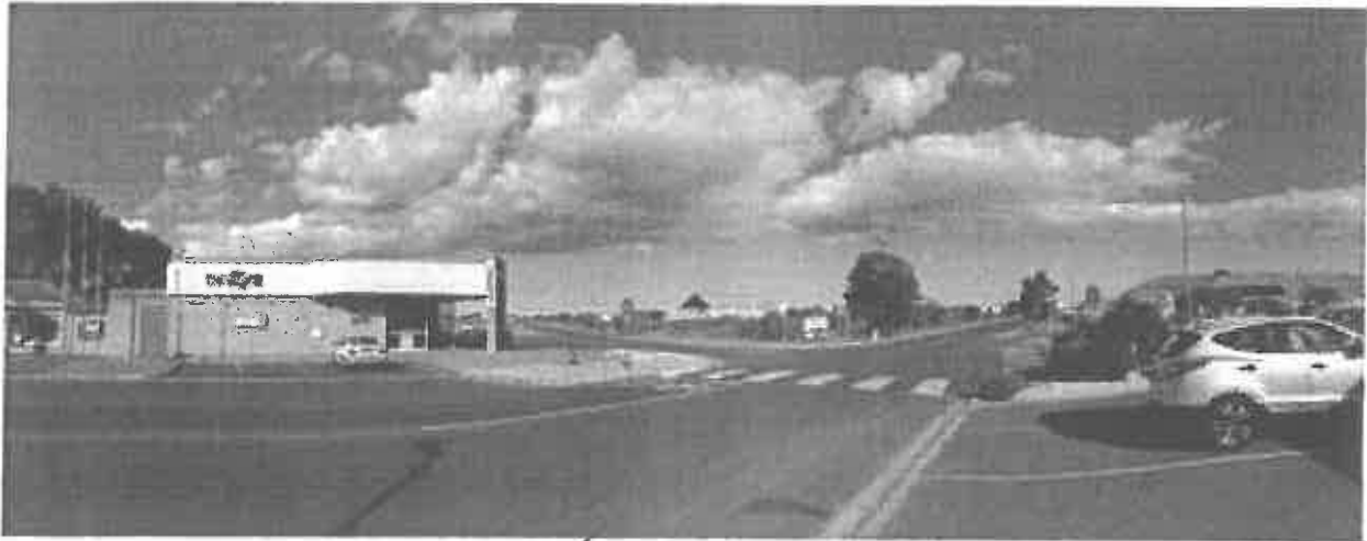
... Photograph 1: Southerly view towards the project site from KOP5.
