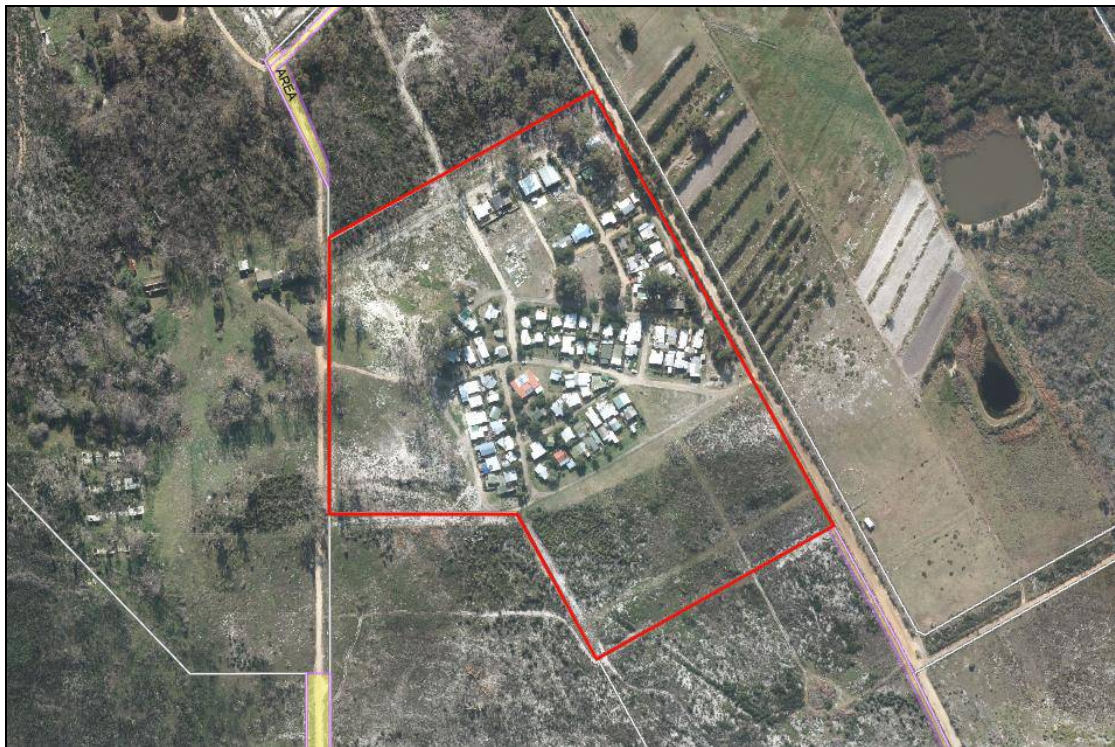
Figure 3: Overstrand Municipality GIS 2020 imagery of Franskraal Caravan Park
