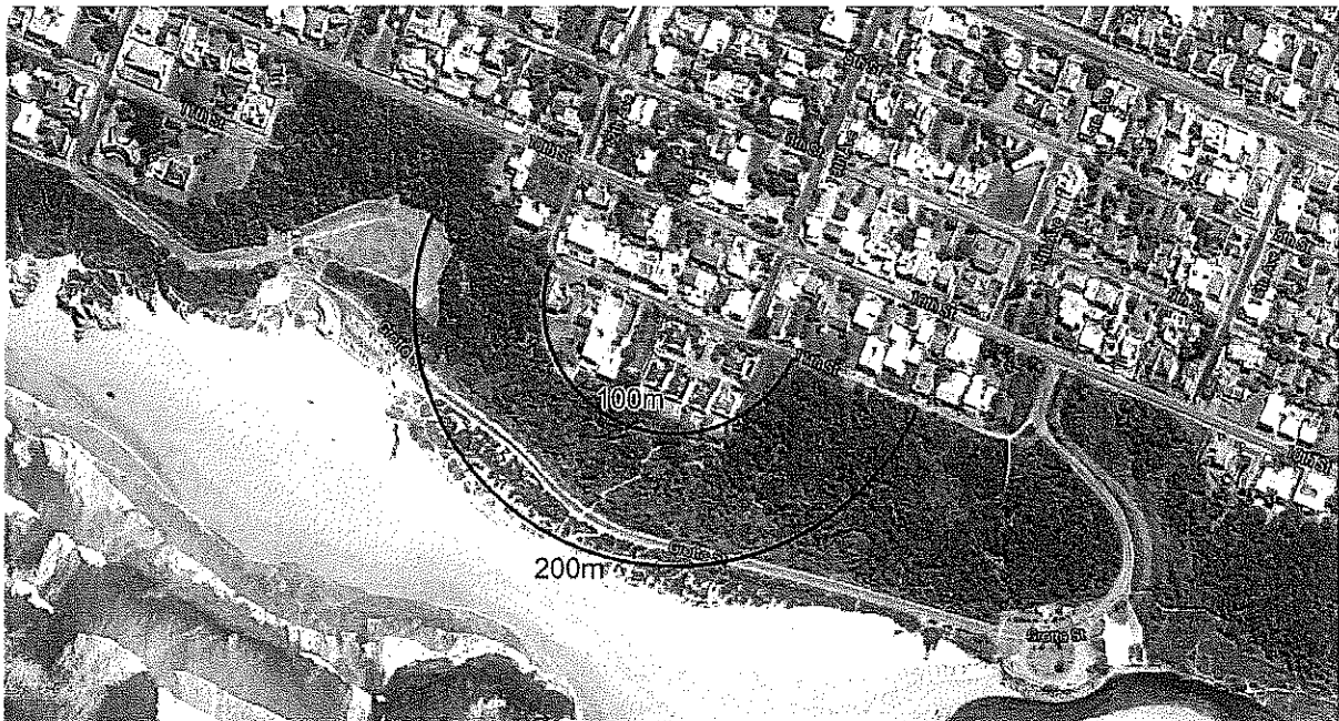
A Google map reflecting the distance of the high water mark from the application site
