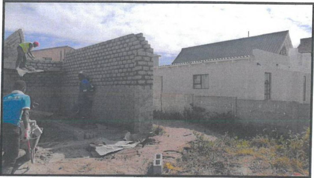
Picture 2: Garage under construction at similar setback as the adjacent dwelling
