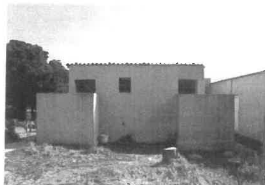
I - Ablutions, looking west (built 1954?) (L.M, 2014)
