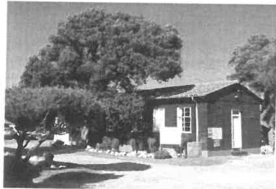
N - "Kliphuis" Conference/ offices/ living unit (built 1942)
