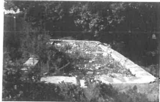
J - Water trough (built 1930's?) (L.M, 2014)
