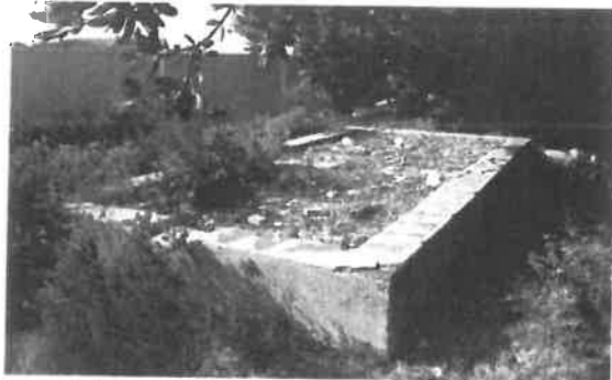
J - Water trough (built 1930's?), looking east (L.M)
