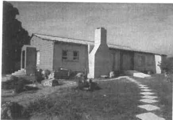
M - Dining/ Functions hall (built 1942/3), looking south-east
