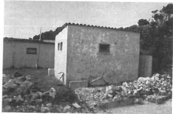
L - Store rooms (built 1954?), looking north (L.M, 2014)
