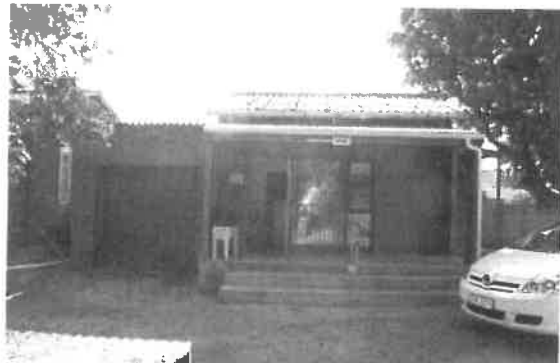
E - Reception (built 1954 ?), looking north (L.M,2014)
