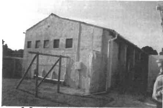
C - Barrack extension (built 2008), looking east (L.Malan)
