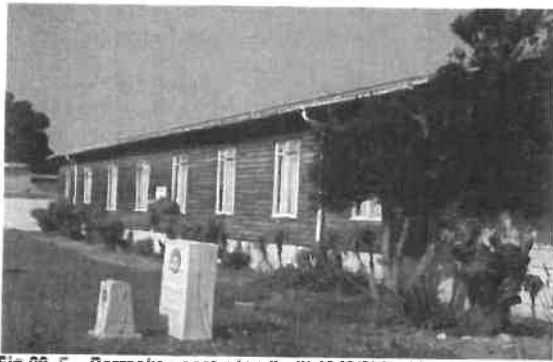
Fig.29 F - Barracks - east wing (built 1942/3),looking n-east (L.M)
