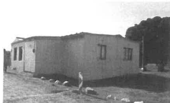
B - Living unit (built 1954 ?), looking north-east (L.Malan)
