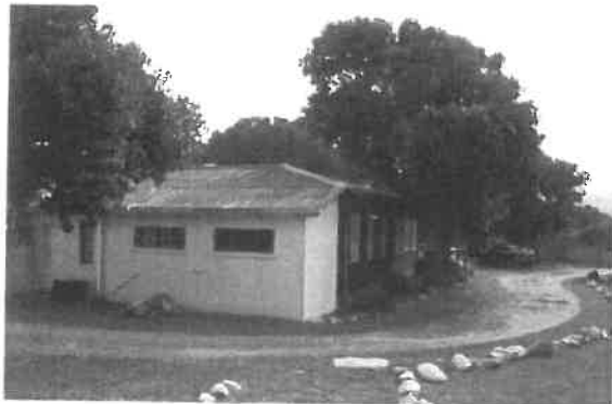
N - "Kliphuis" Conference/ offices/ living unit (built 1942)
