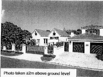
Photo taken ±2m above ground level
