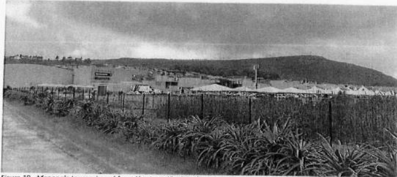
Figure 19 - Monopole tower viewed from Aloe Lane (Option A)
