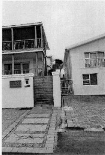
Figure 4: Two metre space between dwellings in 9 th Street.
