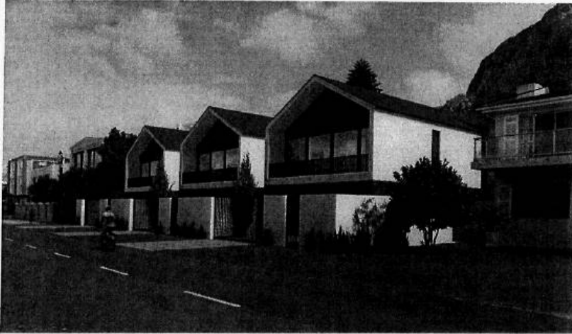
Figure 10: The three new dwellings within the existing streetscape of Tenth Street.
