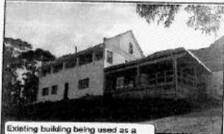
Existing building being used as a water bottling plant on the ground floor. The first floor is being used as accommodation for the manager.
