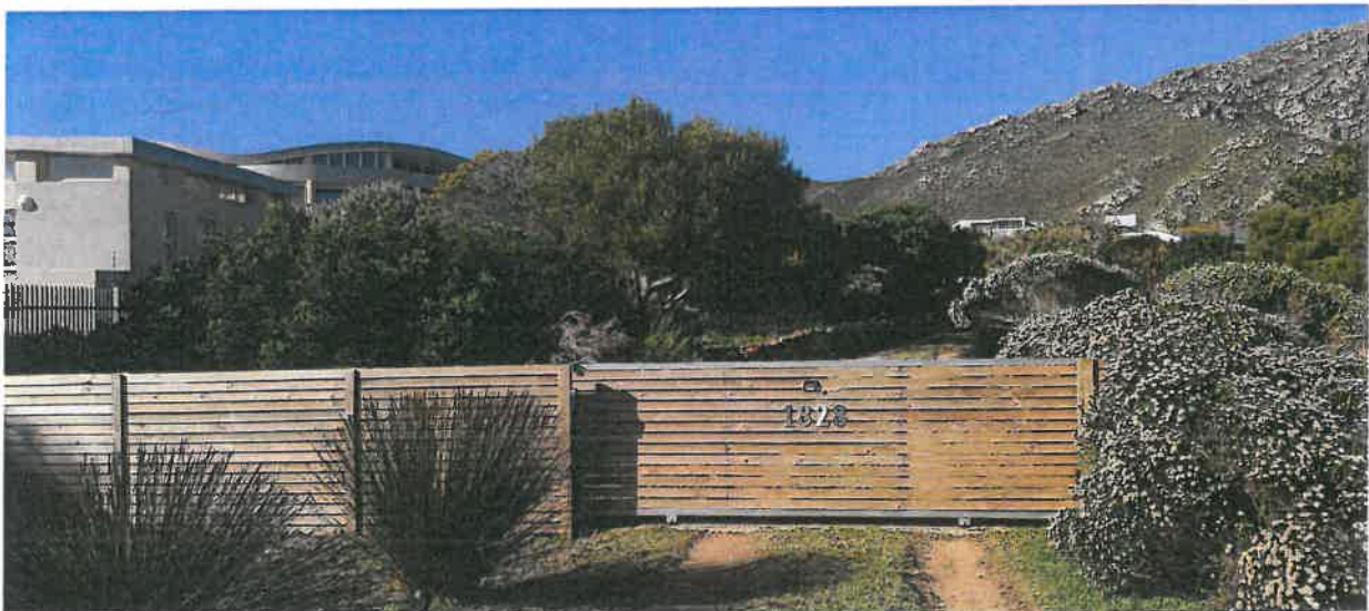
Photo 1: Photo showing existing gate structure in relation to the boundary, as well as the built structures on adjoining Erf 540.
