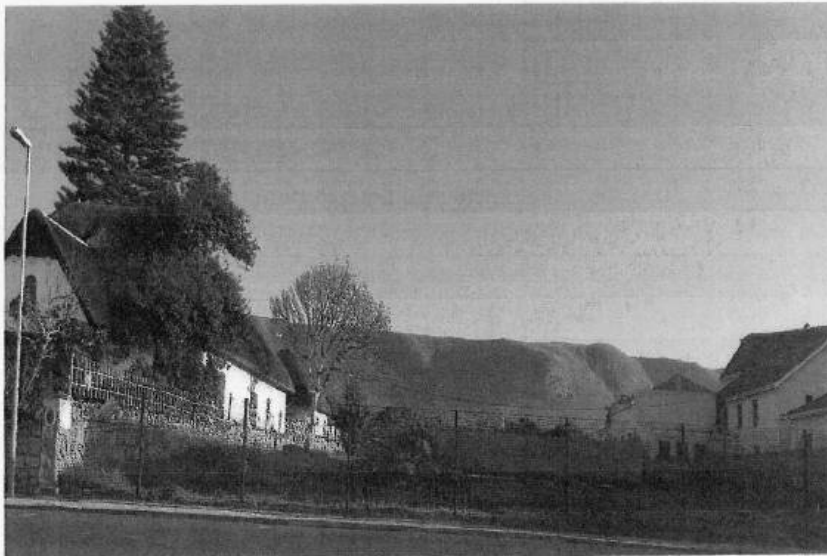
THATCH roofed house (Erf 6127) on boundary of Erf 7182, Marine Drive, Westcliff
