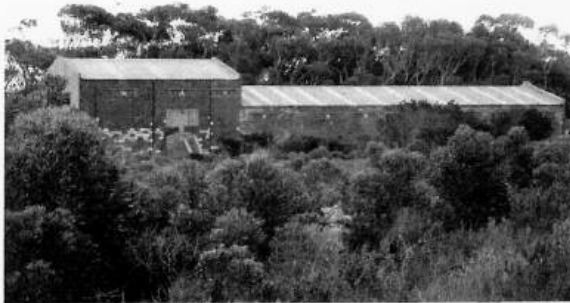
Figure 7: Image taken on 8 May 2021. Building of tasting room and distillery. Clearly in anticipation of a positive outcome.
