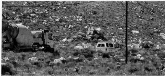
Figure 1 : Trucks and bulldozers using the Rooiels entrance during building operations
