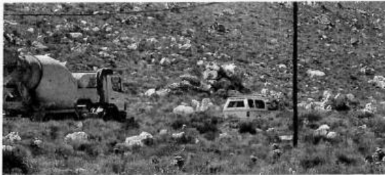
Figure 1 : Trucks and builders using the Rooiels entrance during building operations
