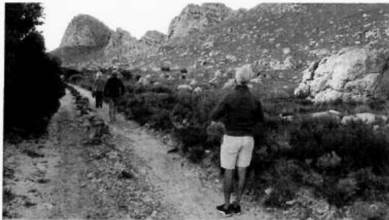
Figure 6: The narrow track to be used by trucks, mini busses and sewerage tankers. No passing places.
