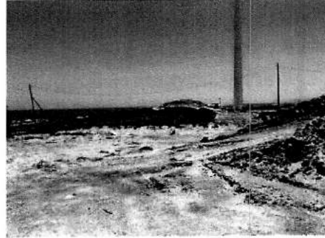
Plate 2. Topsoil stockpiled on site (piles centre and right of image).
