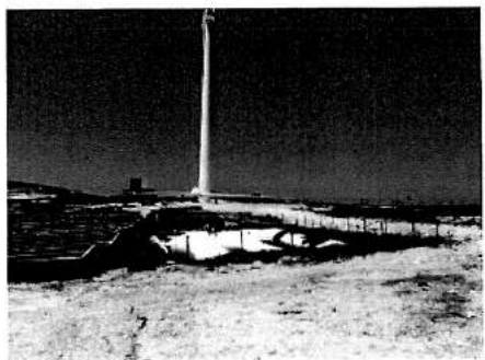
Plate 5. Road to turbine requiring rehabilitation.
