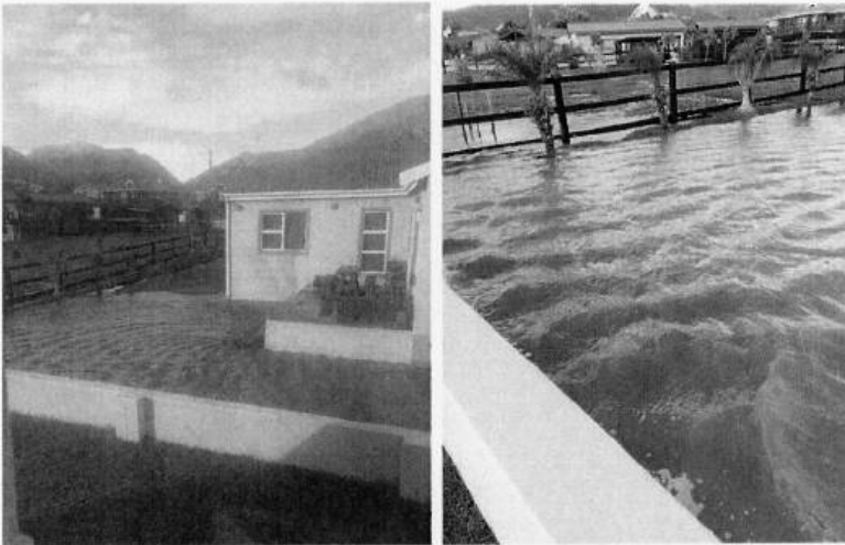
Image of our neighbors (69 Buffels Rd) back-garden due to burst water pipes after flooding in 2021. Image taken from our home by previous owner. The previous owners of our property had to safeguard themselves and built a retainer wall. Our entire property also has a very high water table and it won't take much to cause severe damage.
