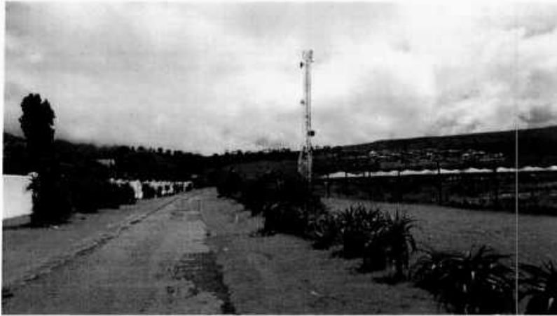
Figure 1: Visual Impression of a Lattice Mast.
