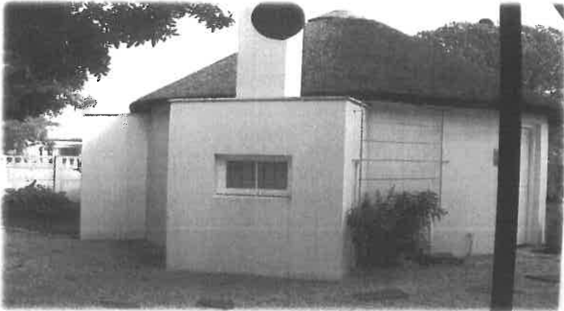
BELOW: EXISTING DETACHED SECOND DWELLING UNIT (RONDAVEL) VIEWED FROM SCHNEIDER STRET
