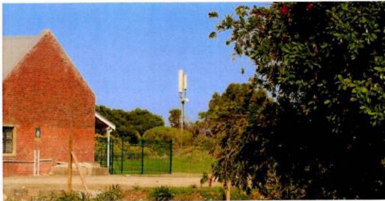
Image 4: Site photo: View from the Main Road looking south east to the temporary TT and proposed site. Source: A de Beer
