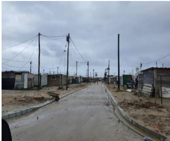
Re-electrification of households in Zwelihle Transit Camp
