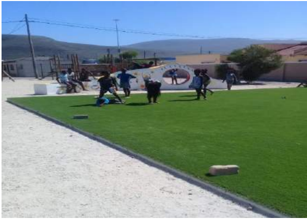
Upgrading of ward 5 play parks (Ilisa Street) (Ward 5)
