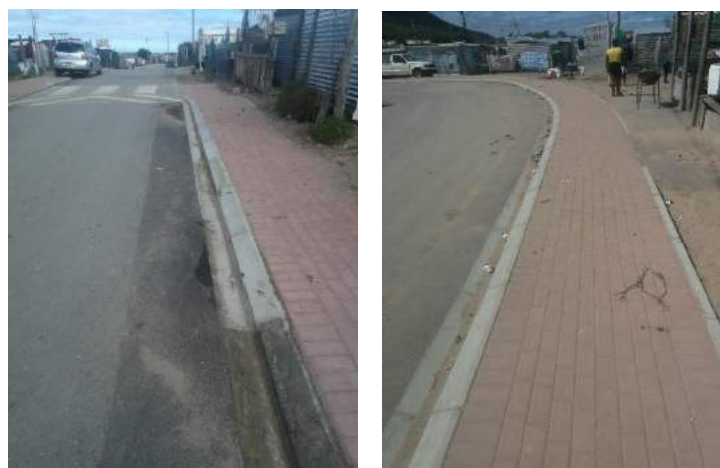
Construction of Sidewalks in Masakhane, Gansbaai (Phase 2)
