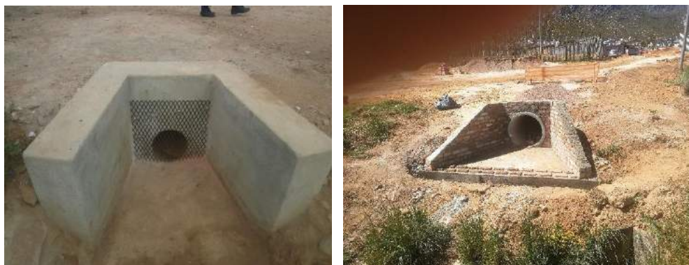
Bulk stormwater infrastructure for Stanford & Masakhane Housing Projects
