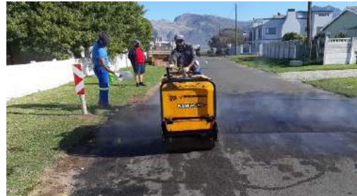
Installation of speed humps in Kleinmond
