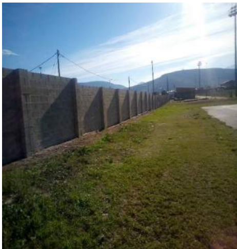
Construction of Z.W Sports Field Boundary Wall (Ward 6)
