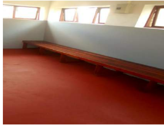
Upgrading of Zwelihle Sport Field Changing Rooms
