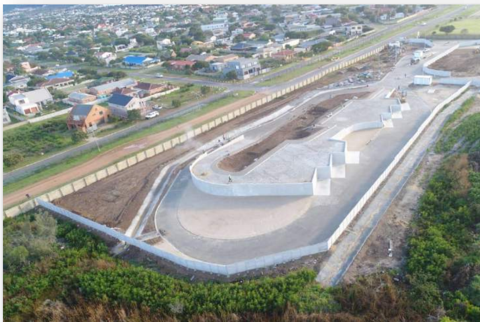
Construction of the New Hermanus public drop-off facility
