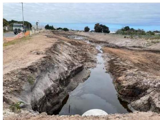
HERMANUS INDUSTRIAL AREA STORMWATER
