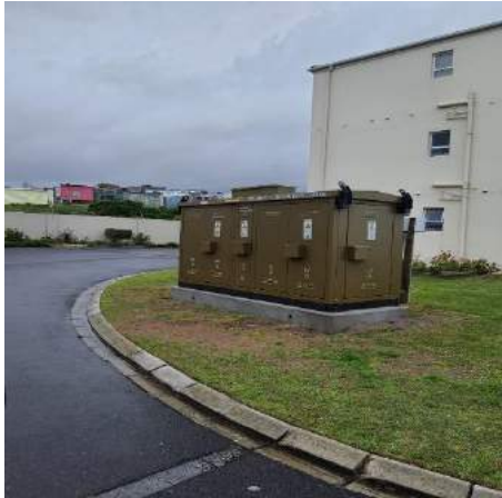
Replacement of miniature substations and installation of new streetlighting in Greater Hermanus
