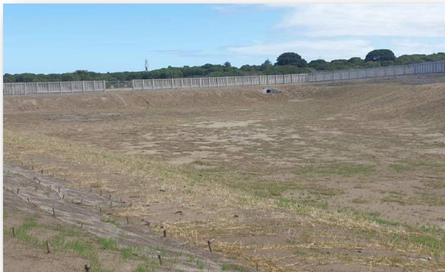
Masakhane Housing Project Stormwater Pond
