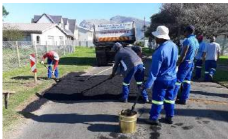
Installation of speed humps in Kleinmond
