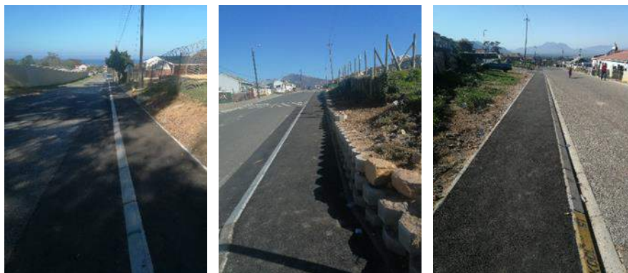
Construction of Sidewalks in Proteadorp, Kleinmond (Phase 2)
