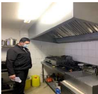
Fire Safety inspections
