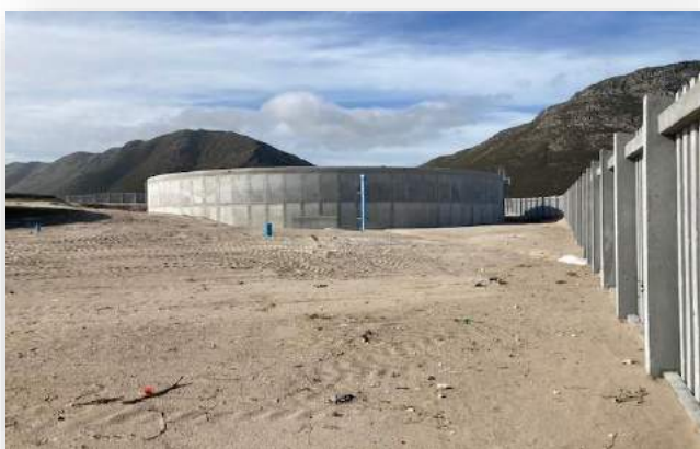
The new 4 Mega litre reservoir constructed at Gansbaai
