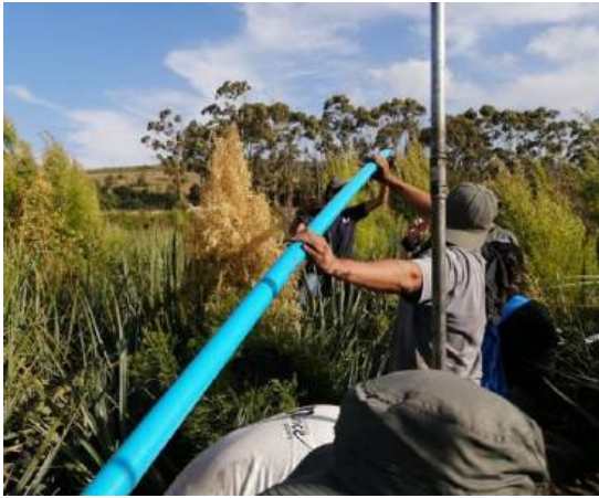
Monitoring wells being installed.
