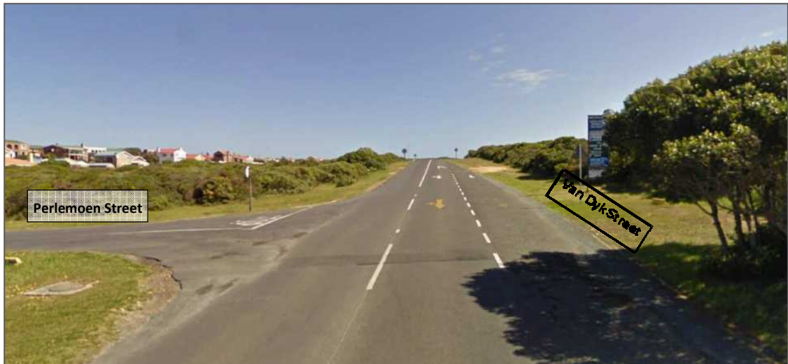
Photo 1: Van Dyk Street / Perlemoen Street intersection. Note the absence of kerbs and stormwater infrastructure
