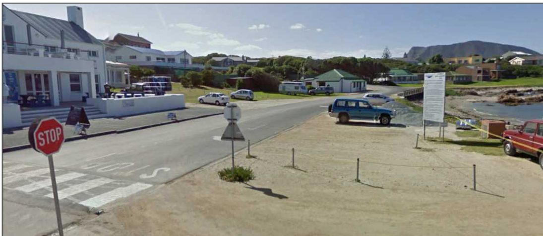
Photo 4: Looking northwards along Kus Drive from Kleinbaai Harbour entrance
