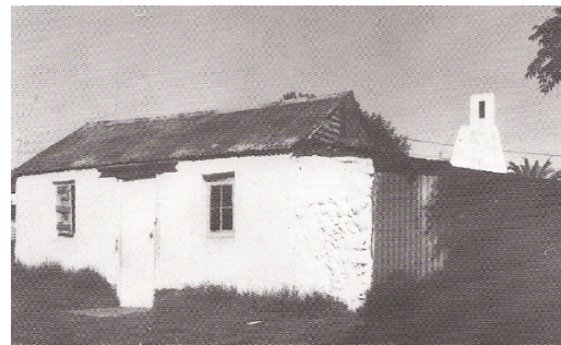
Figure 4: A fisherman's cottage ( palehuis ), Hawston. Corrugated iron kitchen on right added later (In Walton 1995, Andre Pretorius 1994). The structure no longer exists.
