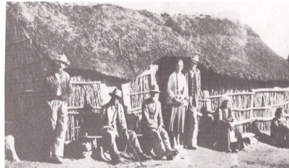
Figure 2: Hawston palehuis (In Walton 1995; Hermanus Old Harbour Museum). The structure no longer exists
