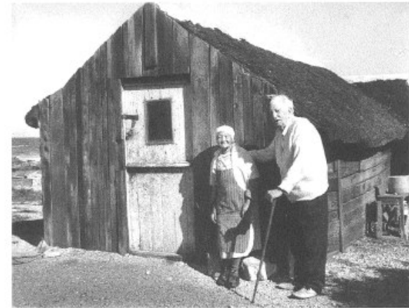
Cottages constructed of timber retrieved from shipwrecks are found in the century-old fishing village of Buffeljagsbaai, between Gansbaai and Struisbaai. James Walton is seen with the owner of one such house, Sophia Swam (André Pretorius 1994).
