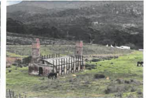
Brick kiln with farm werf below (Scurr 2018)
