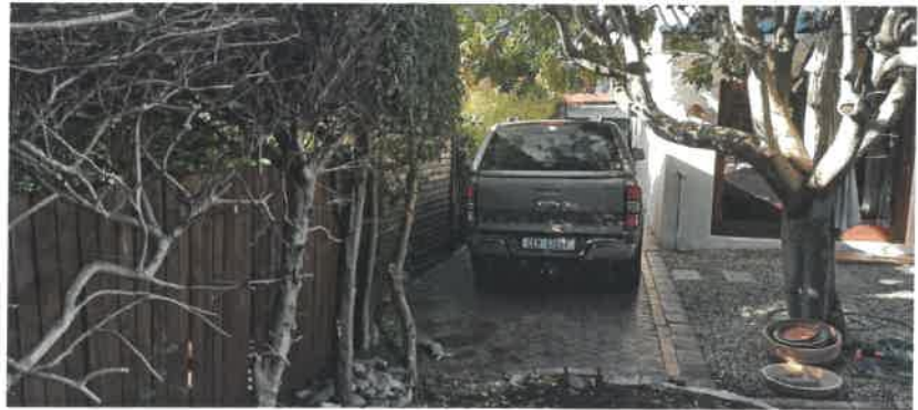
Image 2: Access between existing house & existing boundary wall
