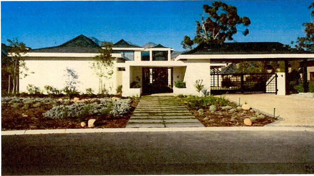
Fig 3. Example presented of roof configuration with double angle. Front and side elevation.
