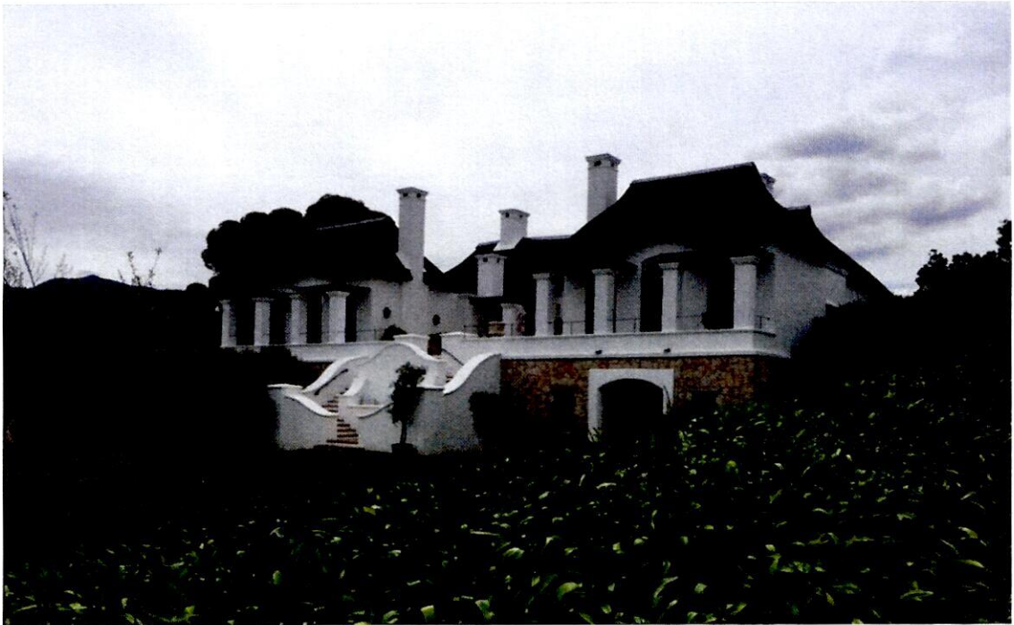
The existing Manor House on the Farm
