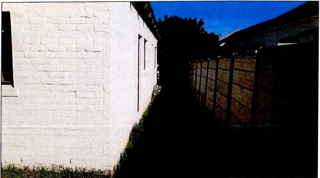
Photo 3: Outbuilding setback of 2m (common boundary building line)
