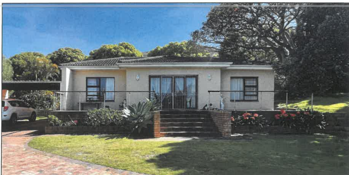
Figure 7: Photographs of the property
