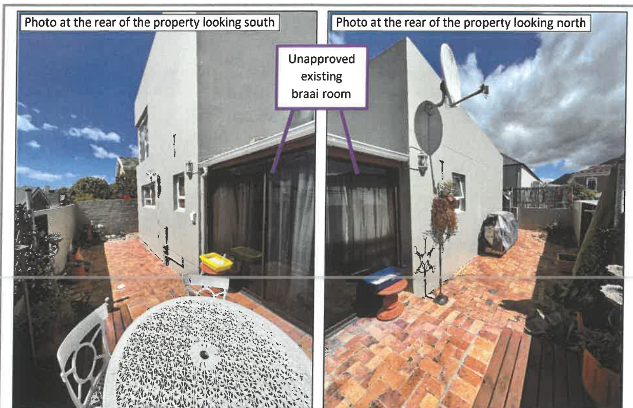
Figure 8: Photographs of the property
