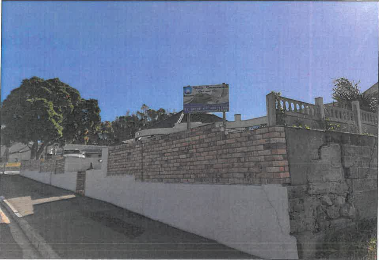
Photo 1. Corner of property on Church Street
