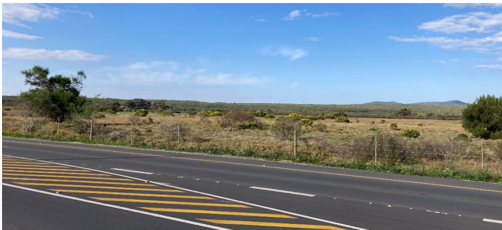
Figure 6: R326 forms the northern boundary of the property
