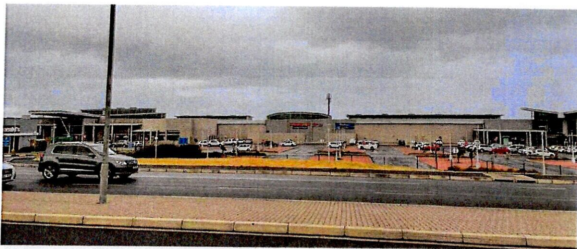
Figure 21 - Monopole tower viewed from the R43 (Option B)
