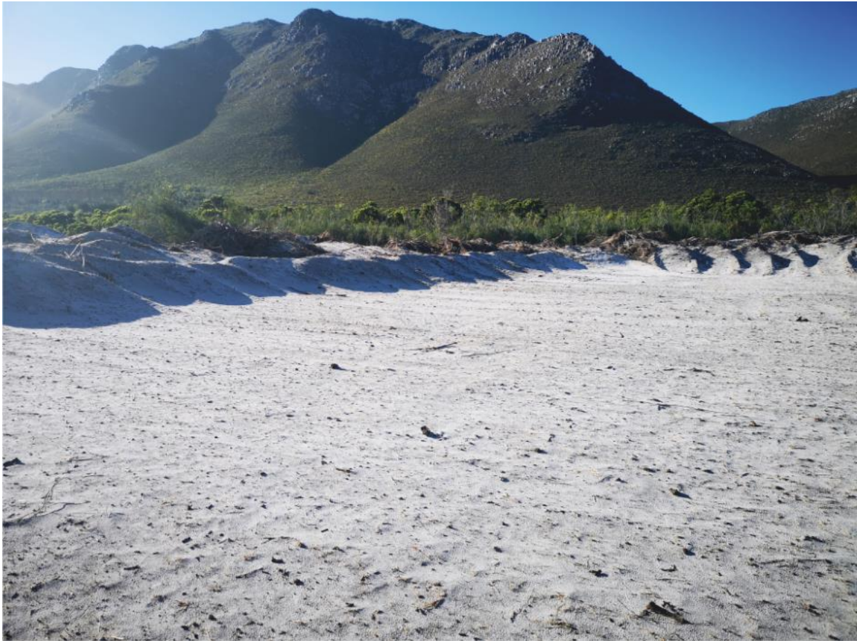
Photo 12: Currently cleared mining block ready for mining. Note the topsoil has been dozed off the affected area along with the vegetation content to perimeter topsoil berms
