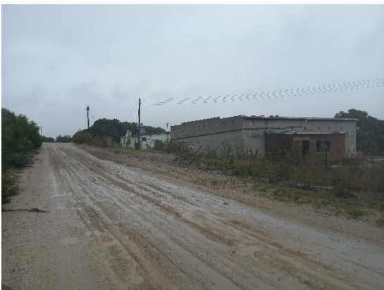
Photo 6: Existing Gravel Access Road and Access to Mine Logistical Area
