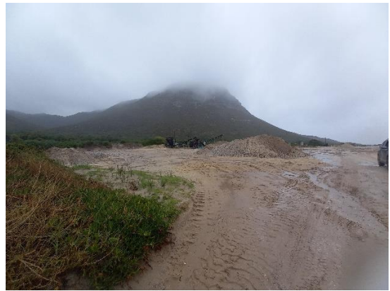
Photo 5: Material Stockpiling and Dispatch Area
