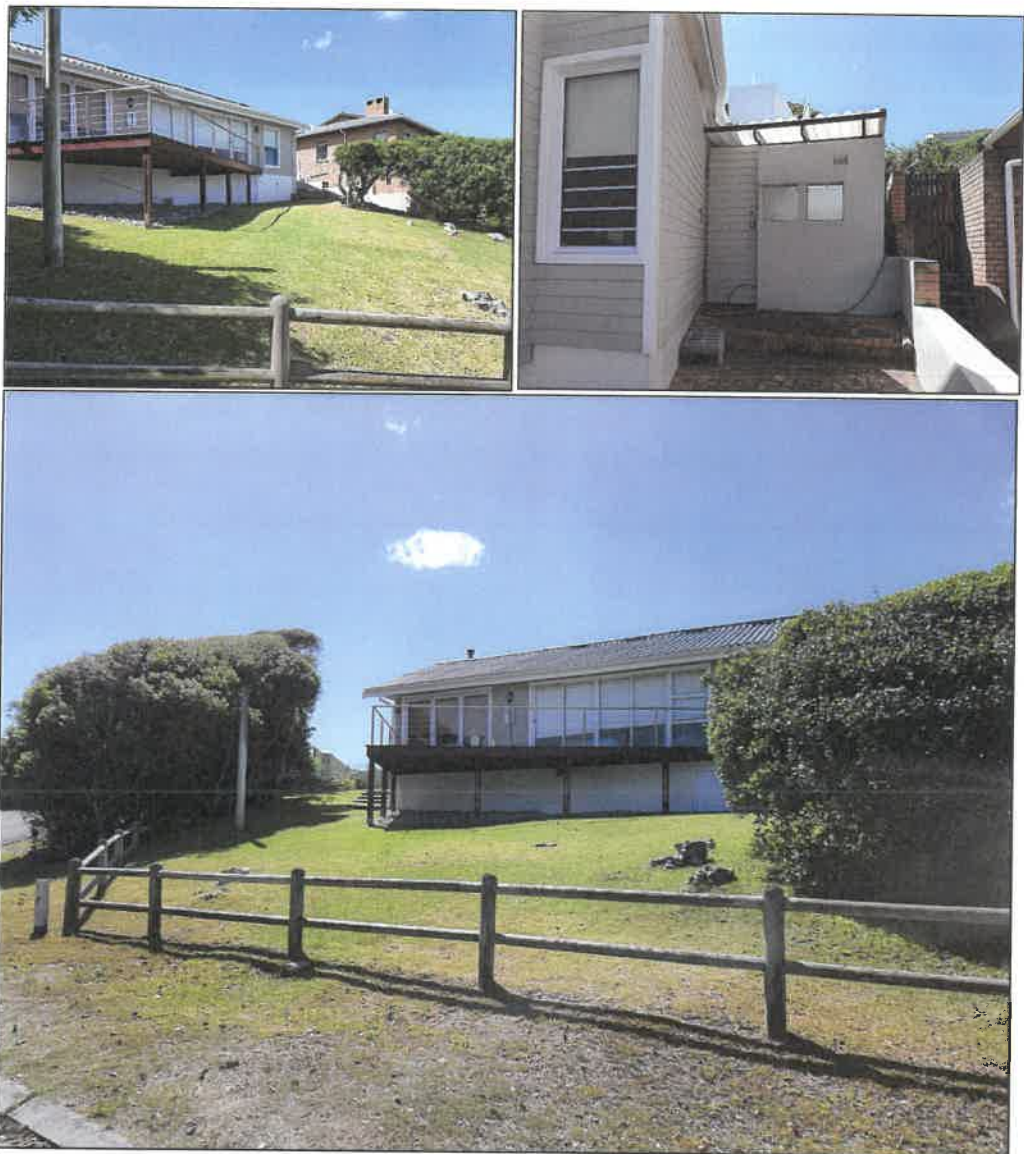
Figure 1: Photographs of the application area
