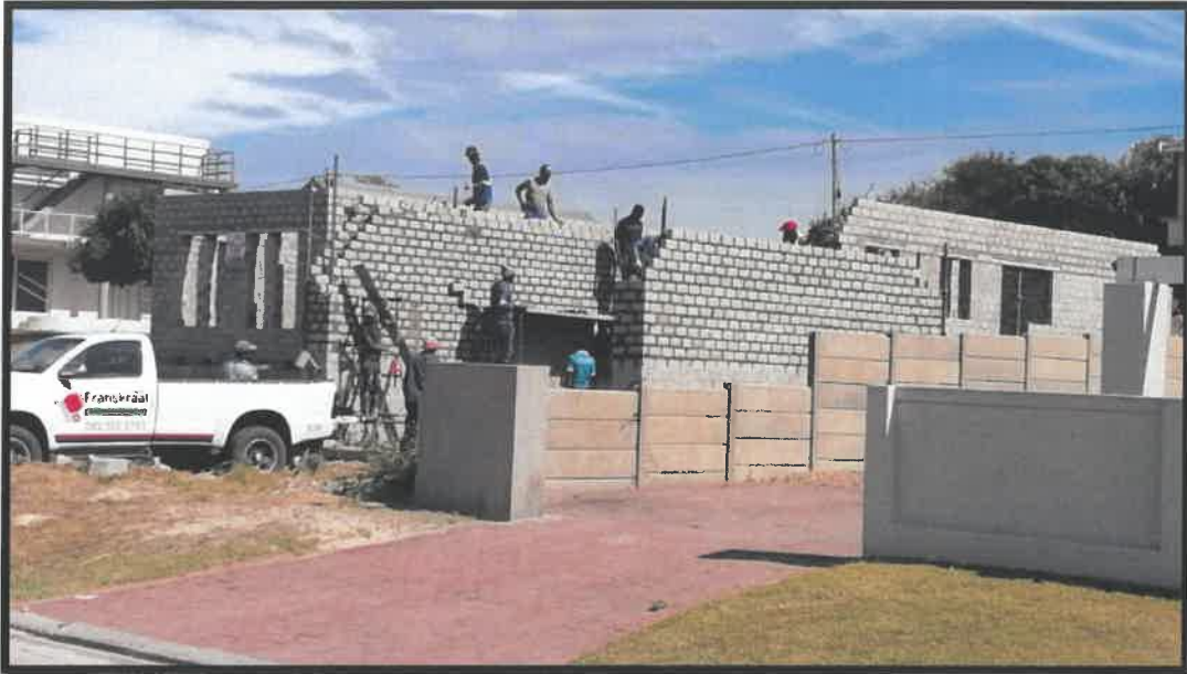
Picture 1: Dwelling under construction as viewed from Naude Street
