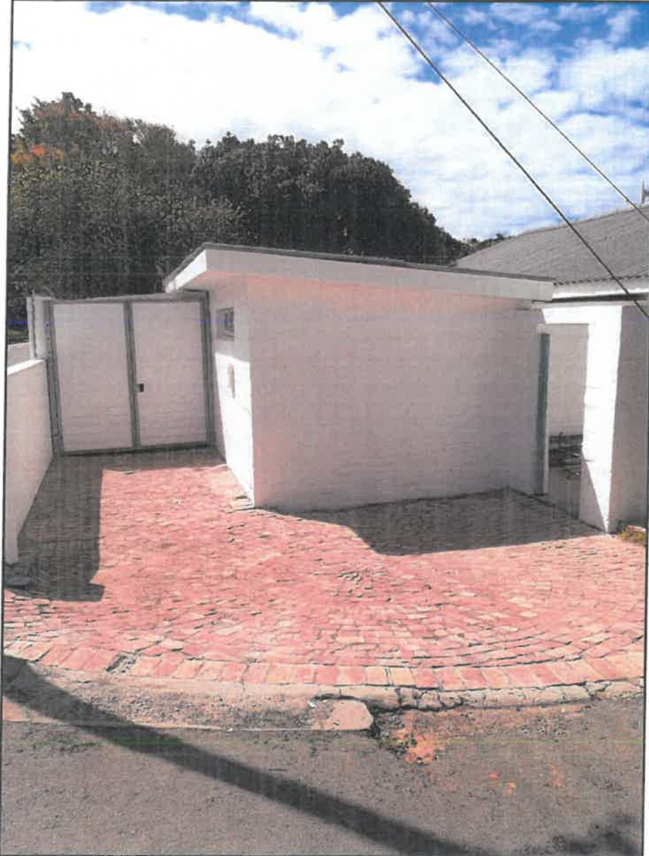
Photo 2: Garage to be converted to bedroom. Ample parking space is available adjacent to the garage.
