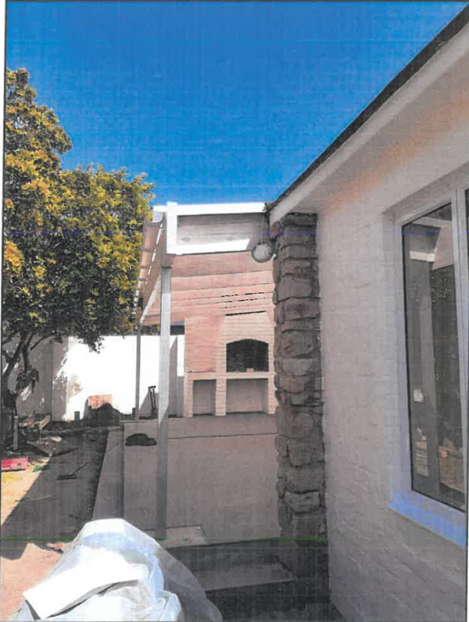
Photo 1: Covered Stoep to be extended
