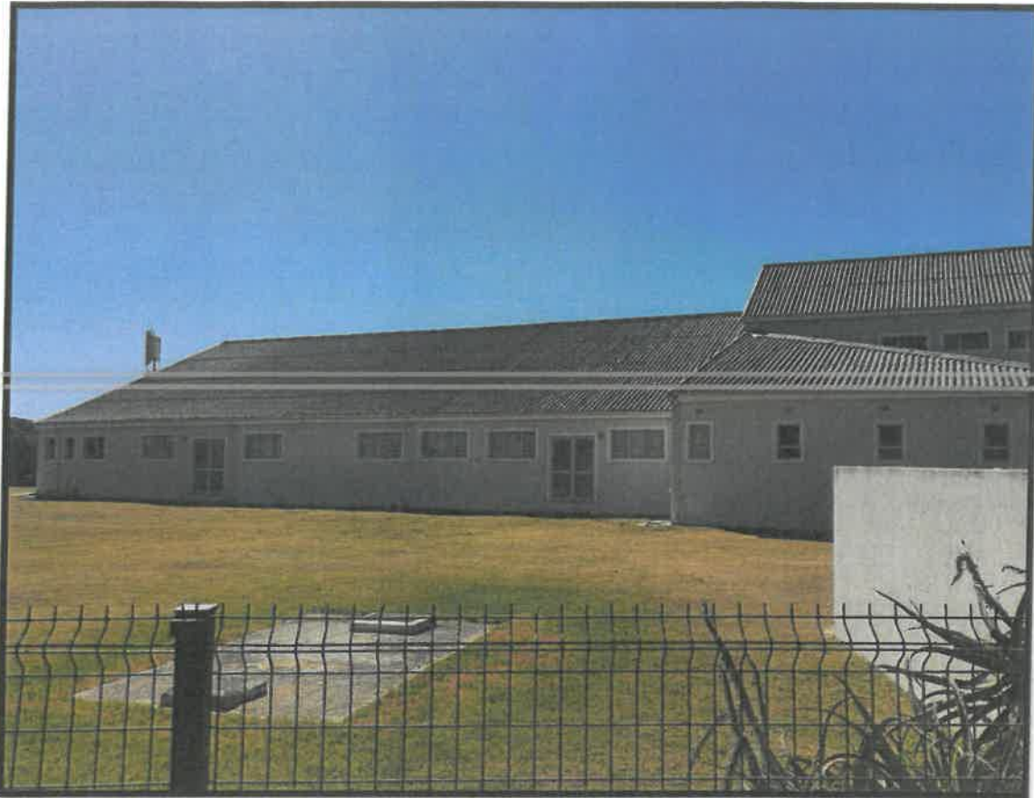
Figure 2 - Photo of the existing transmission apparatus on Erf 2180 Sandbaai
